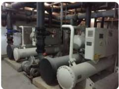
The Ministry of Foreign Affairs Building is located in Dushanbe, Tajikistan. Midea provided the air conditioning solution by adopting water-cooled screw chiller with the total capacity of 1,480kW, and the project was completed in 2012.
